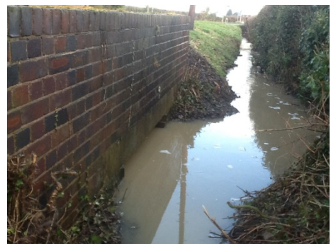
The exit from the culvert in Friday Street
